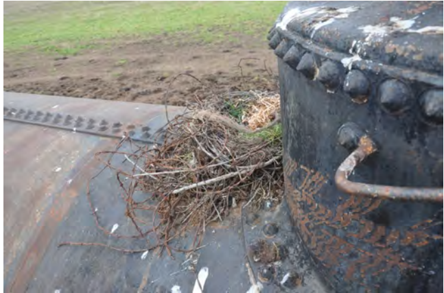
Figure 8. Common Raven nest atop the Hercules Powder tank car.
