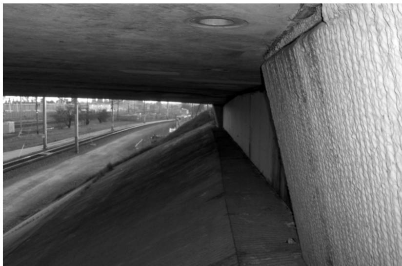
Figure 1. Sloped abutment at west side of the Arden Way overpass of railroad tracks in Sacramento, California. Note weep-hole entrances to bridge nesting chambers in upper foreground. Weep holes here are 0.8 m (2.3 ft) away from the 1.6 m (5 ft) tall vertical abutment wall. One of these holes adjacent to the abutment wall was used in three different years by Northern Rough-winged Swallows.
